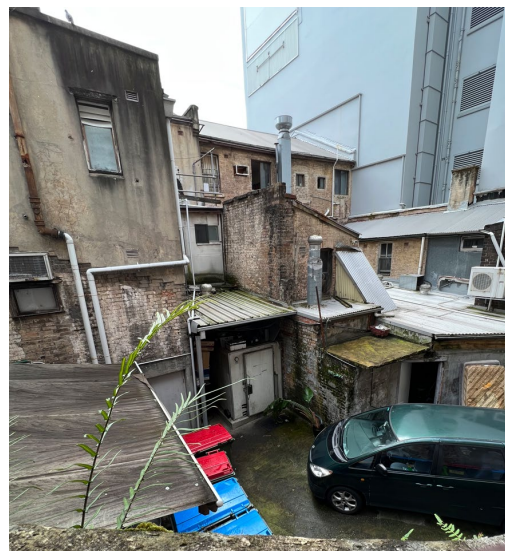
Figure 4-6: Rear of Buildings part 238-40, 232-236 Elizabeth and rear yard from first floor (Source: Curio 2022)
