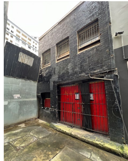
Figure 1-4: Foster Lane (Source: Curio Projects Oct 2022)
