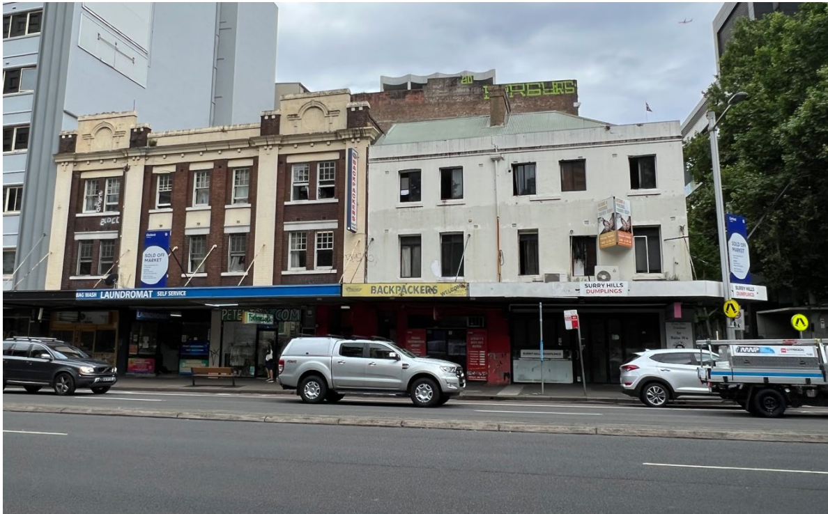
Figure 1-2: Elizabeth Street frontage (Source: Curio Projects Oct 2022)
